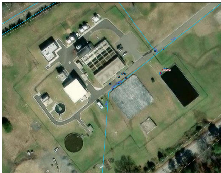
Image: SGWASA Water Treatment Plant
