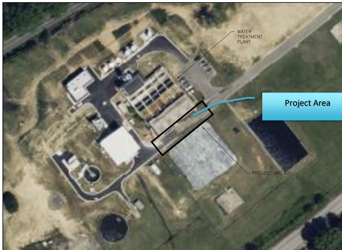
Images: SGWASA Water Treatment Plant – Valve Replacement Project Area.
